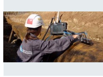
NON DESTRUCTIVE TESTING ON PIPELINE
